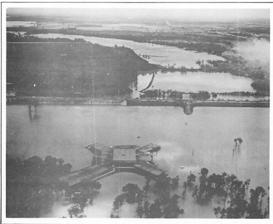
FIGURE I-22. Trinity River flood below Dallas, Texas, April 25, 1957, at Loop 12 highway and River Lake Country Club. Flood reached a 5 foot higher stage at a later date. Photograph by Corps of Engineers, U.S. Army
